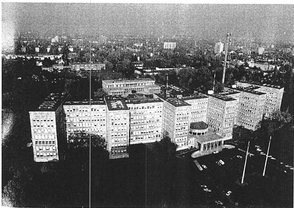
Symbol of power: I.G. Farben was one of the largest corporations in the world and, in a showcase of its power and prestige, its headquarters building was the largest office building in Europe. Within its walls, I.G. executives planned and directed the company's pro-Nazi programs.
